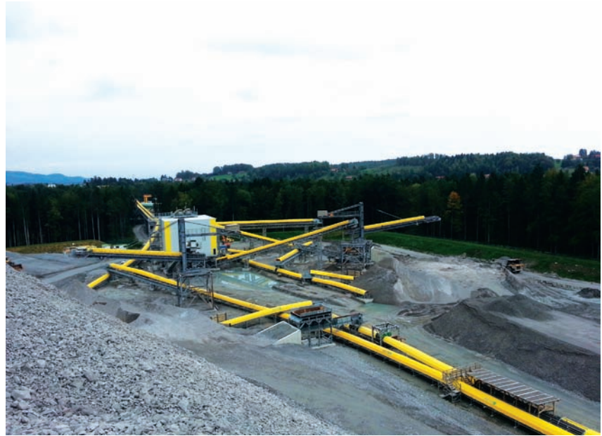
Above: Conveyor setup with temporary storage areas
